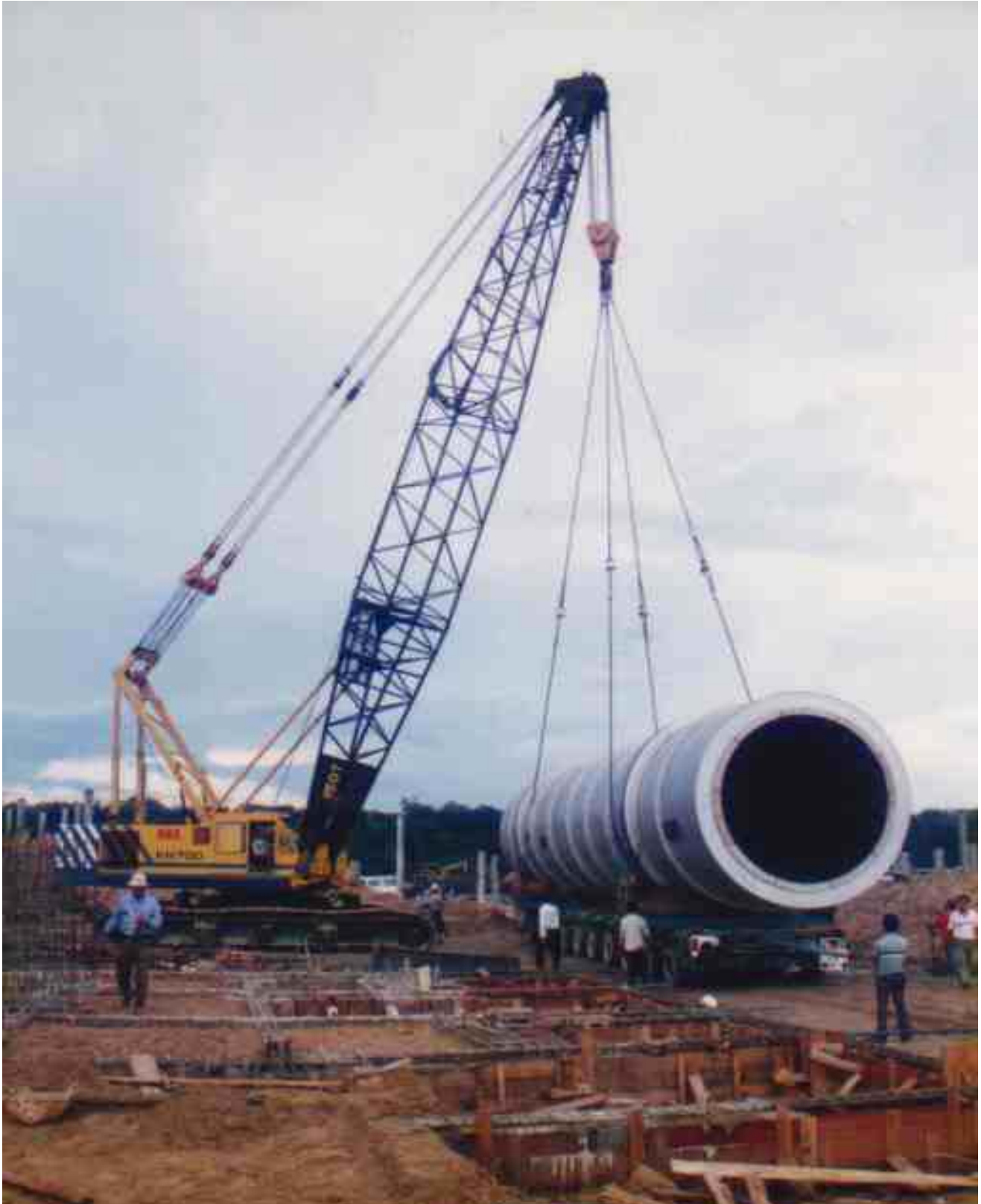
HITACHI KH700 150 tonnes Crawler Crane
