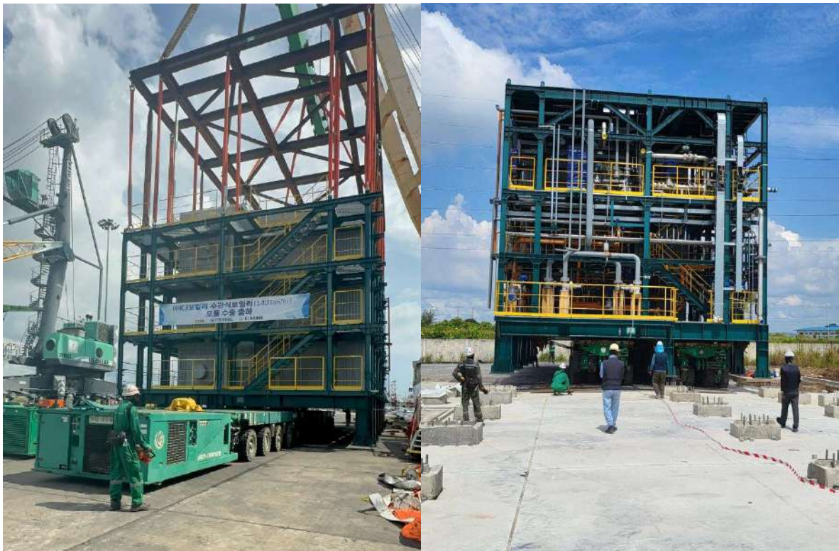
Direct receiving of 290T Boiler (20.5 x 9.96 x 10m) from Crane Vessel onto SCHEUERLE SPMT 12 x 2 (24) axleline + 2 PPU. Transporting from Samalaju Port to OCI MP11 Samalaju Plant and final installation by jacking down onto Site Foundation.
