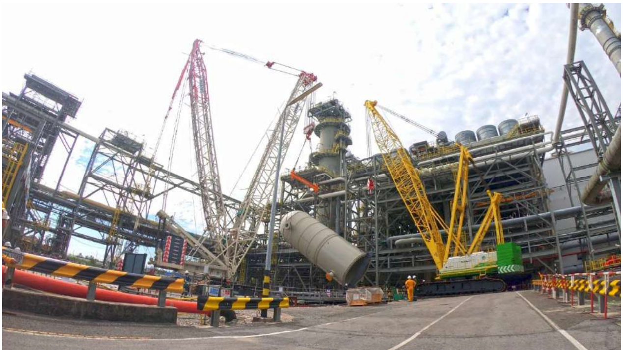
Transportation of Absorber Column from Bintulu Port to MRU Project Site using 10 + ½ PST/THP Goldhofer trailer and lifting utilising Demag CC3800-1
