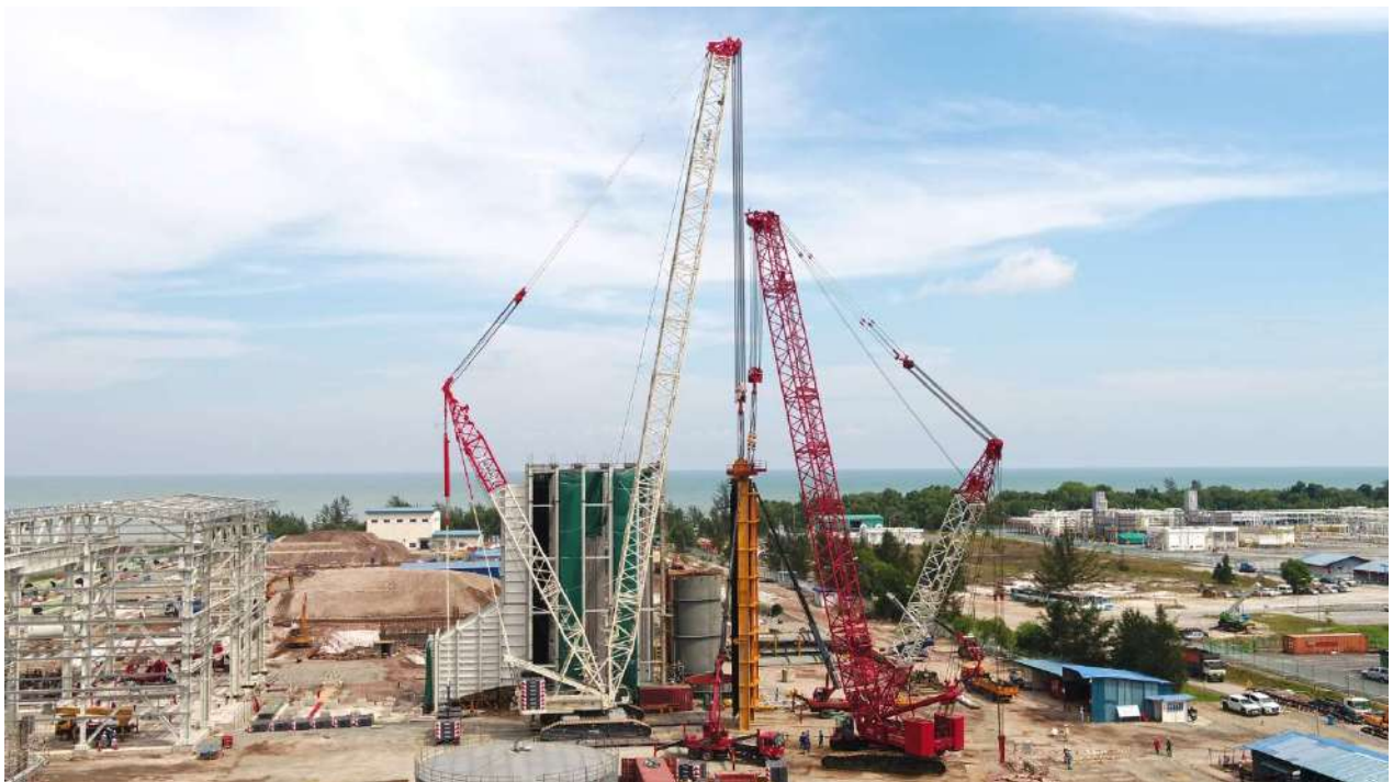
Executing tandem lifting, upending and installation of total 10 units 300 mt HRSG modules for the Tanjung Kidurong Combined Cycle Power Plant Phase 2 project at Bintulu by utilizing 650 mt Demag CC3800-1 and 550 mt Demag CC2600. The job involves non routine critical lifts under complex operations that require additional safety precaution, detail planning and under competent supervision.
