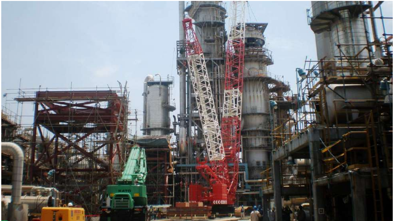
Provision of one (1) unit 600-Ton Demag CC2600 Crawler Crane at Limay, Bataan, Philippines for lifting one (1) unit Cyclone Assembly weighing 165 MT, with dimension of 7.6m(D) X 12m(H) and lifting height of 55m at Petron Refinery.
