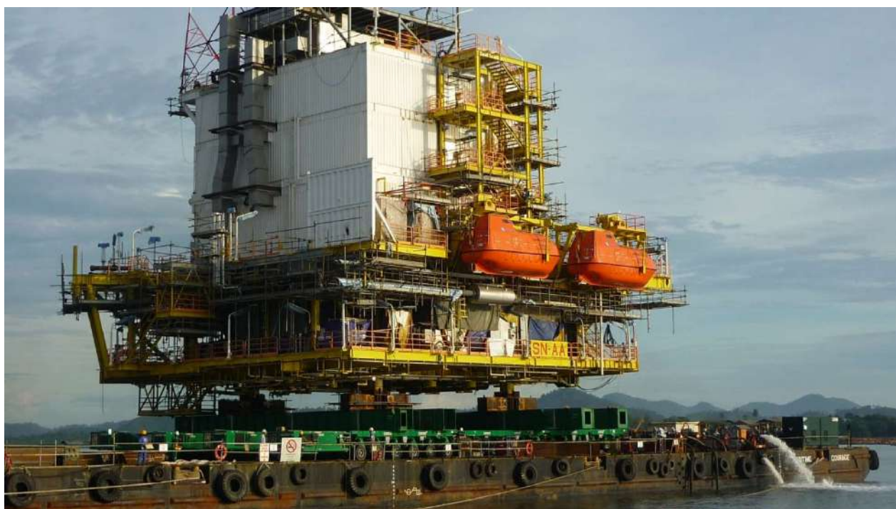
Shifting and loadout of SN-AA LQ Topside with combined weight of approximately 1900MT from fabrication site onto barge in April 2013 for our esteemed client, Kencana HL Sdn Bhd. For SN-AA LQ Topside's shifting and loadout, we utilized our Scheuerle's 72 axelines Self-Propelled Modular Transporter (SPMT) with 4 power packs. Combination of Scheuerle and Goldhofer's 120 axelines SPMT with 5 powerpacks is utilized for the shifting and loadout of SN-PA CPP Topside.
