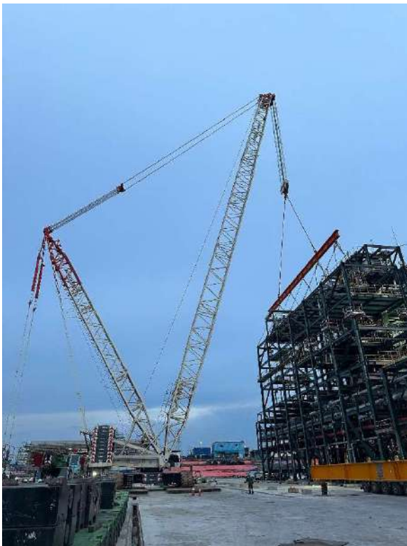
Transportation of 184T Module from Samalaju Port to OCI ME1 Samalaju Plant utilising SCHEUERLE SPMT 30 x 2 (60) axeline and 2 PPU. Using 800T DEMAG CC3800-1 with Boom Booster lifting Module + Accessories with a total load of 282T on top of another Module for the final installation.
