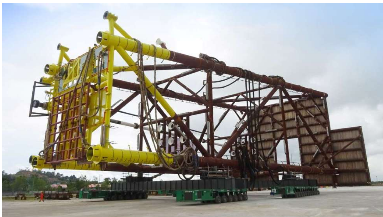
Shifting of 766Te BP-A (Bunga Pakma – A) Jacket by utilising our 36 axelines of Scheuerle 4th Gen. Self Propelled Modular Trailers (SPMT's) coupled with 4units hydraulic Powerpack units from the fabrication area to the quayside for our prestigious and distinguished clients Oceanmight Sdn Bhd on the 16th of August 2017, at their fabrication yard in Kuching, Sarawak, for Repsol Oil & Gas Malaysia Ltd. The synchronised shifting operation lasted for around one hour and subsequently upon reaching the quay side, the Jacket was loaded out to the already pre-ballasted 330' flat top ballastable barge by utilising 20nos of our diesel driven ballast pumps.
