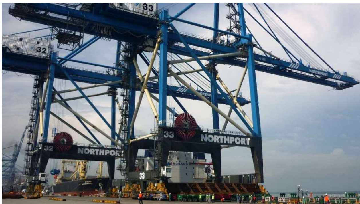
Load-in operations in May 2013 for 2 units of 55 Ton STS Dong Bang Quay Cranes from barge "Dongbang Giant No. 3" to Northport Wharf No. 17 for our esteemed client, ALE Heavylift (M) Sdn. Bhd. utilizing our Scheuerle 128 axle-lines with 4 powerpacks at Northport, Klang.
