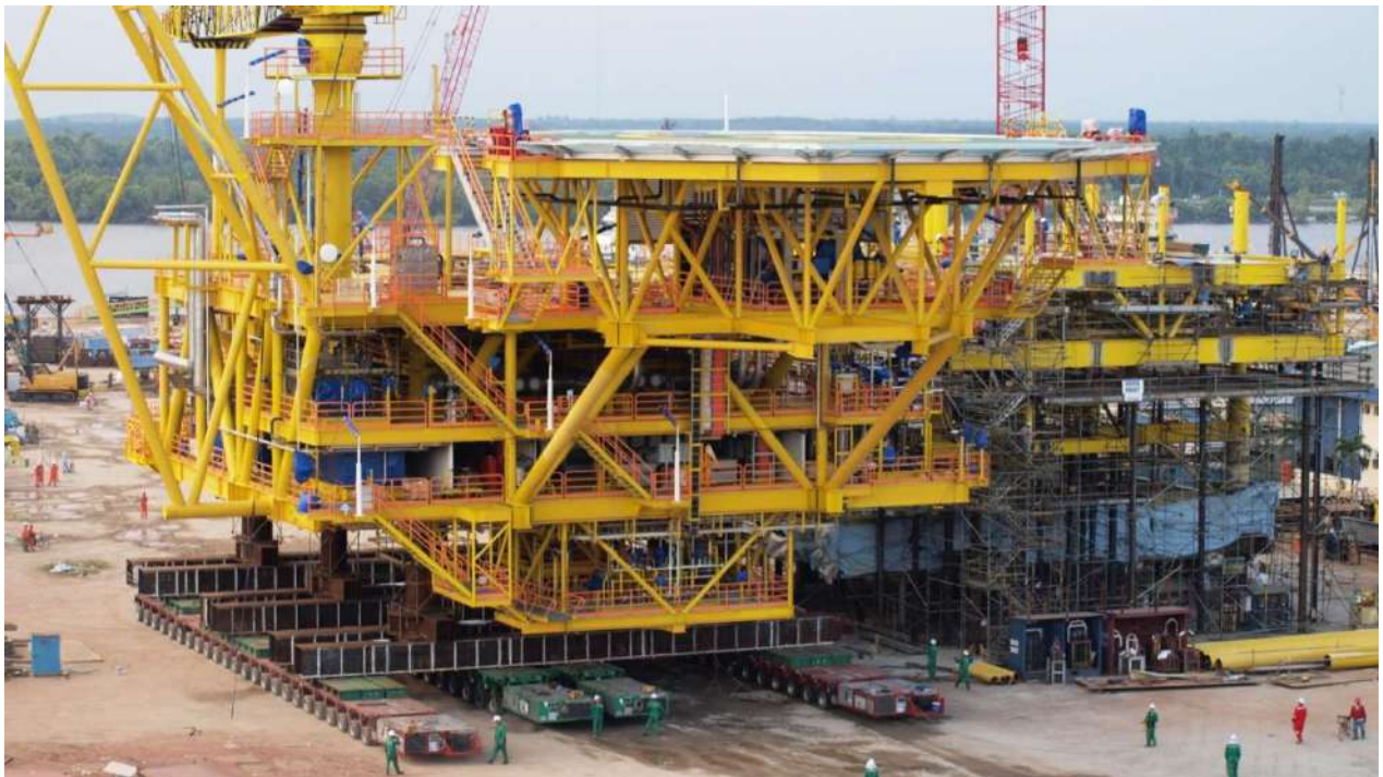
Shifting and Loadout of F28 DR-A TOPSIDE at Kencana HL Yard, Lumut; a project by Shell Berhad, on 21st-22nd June 2011. A total of 2 x 24 axles SLE and 2 x 12 axles ESE (72 axles Goldhofer trailers) were used to transport the topside weighing almost 2224 tonnes. The topside was shifted at a distance of 400 meters before crossing over to the barge the following day. 14 ballast pumps were used for ballasting.
