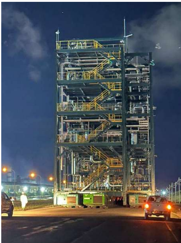
Load-in operation of 826T Module (L38 x W12 x H34m) from Samalaju Port to OCI ME1 Samalaju Plant utilising SCHEUERLE SPMT 36 x 3 (108) axeline and 3 PPU. The final installation is completed by jacking down onto Site Foundation through Gen 4 SCHEUERLE wireless remote system ensuring precision control.
