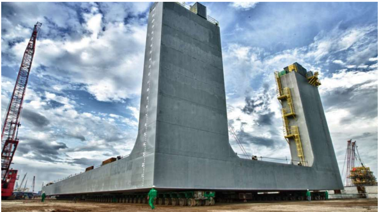
Shifting, Load Out and Barge Ballasting of Dockwise's Buoyancy Tank with combined weight of 4300MT utilizing 168 axle-lines Goldhofer Self-Propelled Modular Transporter at Kencana Petroleum's Yard, Lumut, Perak, Malaysia. After which, a separate operation of Load In, Shifting and Barge Ballasting is being carried out using the same equipments at Malaysian Marine & Heavy Engineering's Yard, Pasir Gudang, Johor, Malaysia
