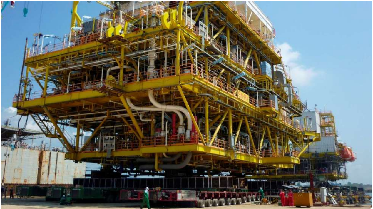
Shifting and loadout of SN-PA CPP Topside with combined weight of 3400MT from fabrication site onto barge in April 2013 for our esteemed client, Kencana HL Sdn Bhd at Lumut, Perak utilizing our Scheuerle & Goldhofer 120 axle-lines with 5 powerpacks.
