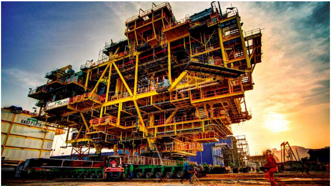
Shifting, Weighing, Load Out and Barge Ballasting for Newfield Peninsula Malaysia INC's CPP Topside with combined weight of 3500MT utilizing 120 axle-lines Goldhofer Self-Propelled Modular Transporter.
