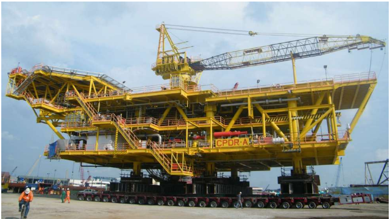
Shifting and loadout of CPDR-A Topside weighing 1958 MT for Cili Padi Gas Field Development Project at Kencana Yard, Lumut utilizing 72 axles Goldhofer PST-SLE and PST-ESE Electronic Multiway Steering System Modular Transporter on the 19th September 2010. Ten (10) units of ballast pump were used on the offshore barge to maintain stability during the cross-over.
