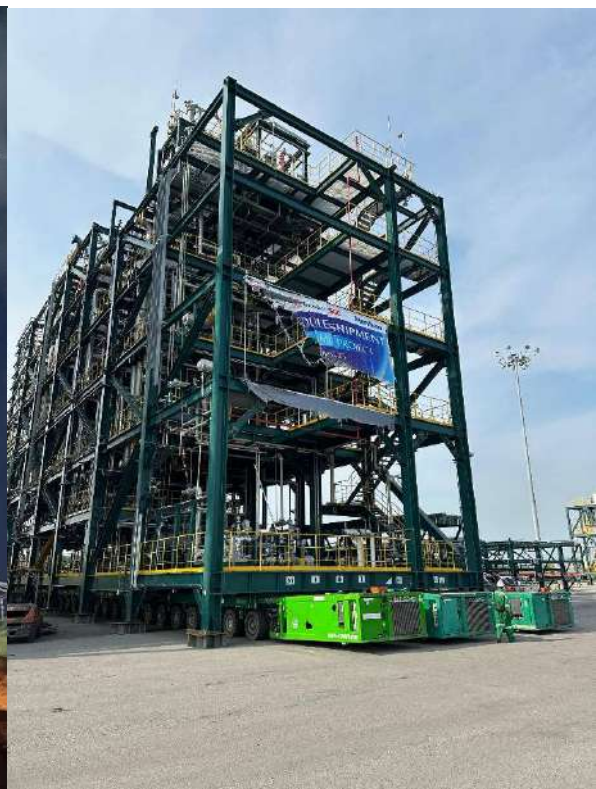
Load-in operation of 826T Module (L38 x W12 x H34m) from Samalaju Port to OCI ME1 Samalaju Plant utilising SCHEUERLE SPMT 36 x 3 (108) axeline and 3 PPU. The final installation is completed by jacking down onto Site Foundation through Gen 4 SCHEUERLE wireless remote system ensuring precision control.
