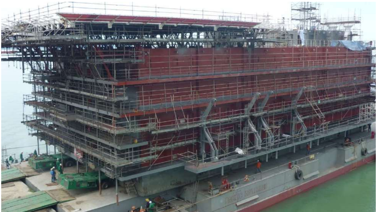
Shifting and Load out of a 2000 MT Accommodation Unit (H-131) onto a 111m Accommodation Barge in Boustead Penang Shipyard (BPS), Pulau Jelajak, Penang on 21 May 2011. A total of 2 x 36 - axle lines single file of Goldhofer THP combined with PST Self Propelled Hydraulic Controlled Modular Transporter.
