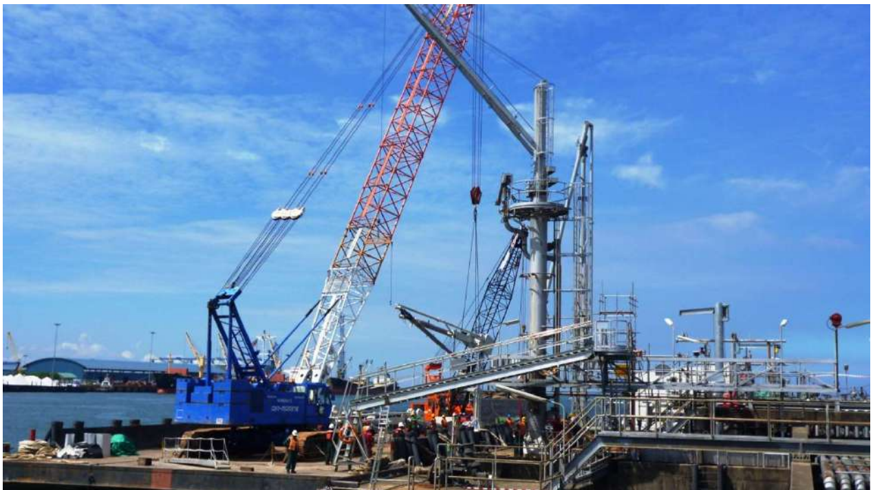
Erection of Sarawak SHELL Berhad's Loading Arm weighing 50 MT utilizing Hitachi KH500 as main crane and Kobelco 7450 as tailing crane.
