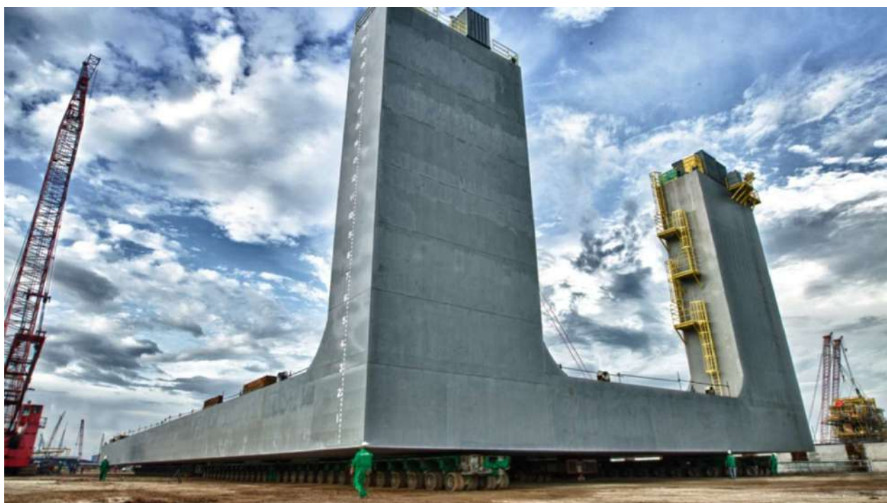
Shifting, Load Out and Barge Ballasting of Dockwise's Buoyancy Tank with combined weight of 4300MT utilizing 168 axle-lines Goldhofer Self-Propelled Modular Transporter at Kencana Petroleum's Yard, Lumut, Perak, Malaysia. After which, a separate operation of Load In, Shifting and Barge Ballasting is being carried out using the same equipments at Malaysian Marine & Heavy Engineering's Yard, Pasir Gudang, Johor, Malaysia
