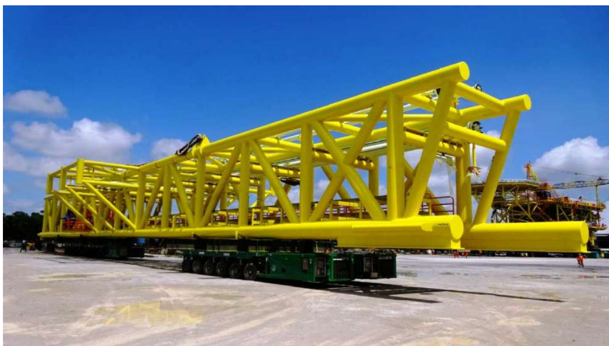
Shifting of 393Te KNDW-D Bridge by utilising our 24 axelines of Scheuerle 4th Gen. Self Propelled Modular Trailers (SPMT's) coupled with 2units hydraulic Powerpack units from the fabrication area to the quayside for our prestigious and distinguished clients Oceanmight Sdn Bhd on the 26th of May 2017, at their fabrication yard in Kuching, Sarawak, for Repsol Oil & Gas Malaysia Ltd. The synchronised shifting operation lasted for around one hour and subsequently upon reaching the quay side, the Bridge was loaded out to the already pre-ballasted 330' flat top ballastable barge by utilising 18nos of our diesel driven ballast pumps.
