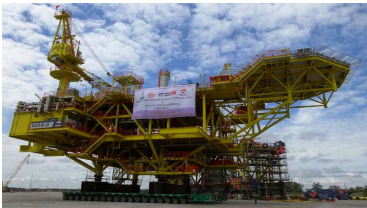
Shifting of 1756Te KNDW-D Topside by utilising our 72 axelines of Scheuerle 4th Gen. Self Propelled Modular Trailers (SPMT's) coupled with 4units hydraulic Powerpack units from the fabrication area to the quayside for our prestigious and distinguished clients Oceanmight Sdn Bhd on the 28th of May 2017, at their fabrication yard in Kuching, Sarawak, for Repsol Oil & Gas Malaysia Ltd. The synchronised shifting operation lasted for around two hours and subsequently upon reaching the quay side, the Topside was loaded out to the already pre-ballasted 330' flat top ballastable barge by utilising 18nos of our diesel driven ballast pumps.
