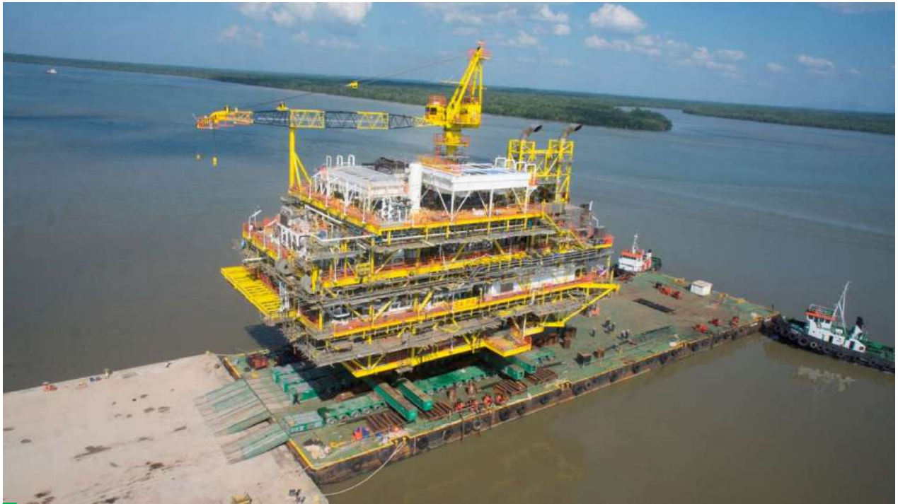
✓ The SA-PA Topside weighing 2408MT was fabricated at BDEWC yard in Kuching, Sarawak for Murphy Sarawak Oil Co. Ltd. AIR-MARINE utilised 96 axle lines of Self-Propelled Modular Trailers and 4 power packs to transport and loadout the structure to barge 'Maritime Courage'. 16 units of deck pumps were used for the ballasting / deballasting works during the loadout. AIR-MARINE also provided 4x27m loadout beams, 15 units of RO-RO Ramps and 30 units of wooden wedges required for the loadout operation.
