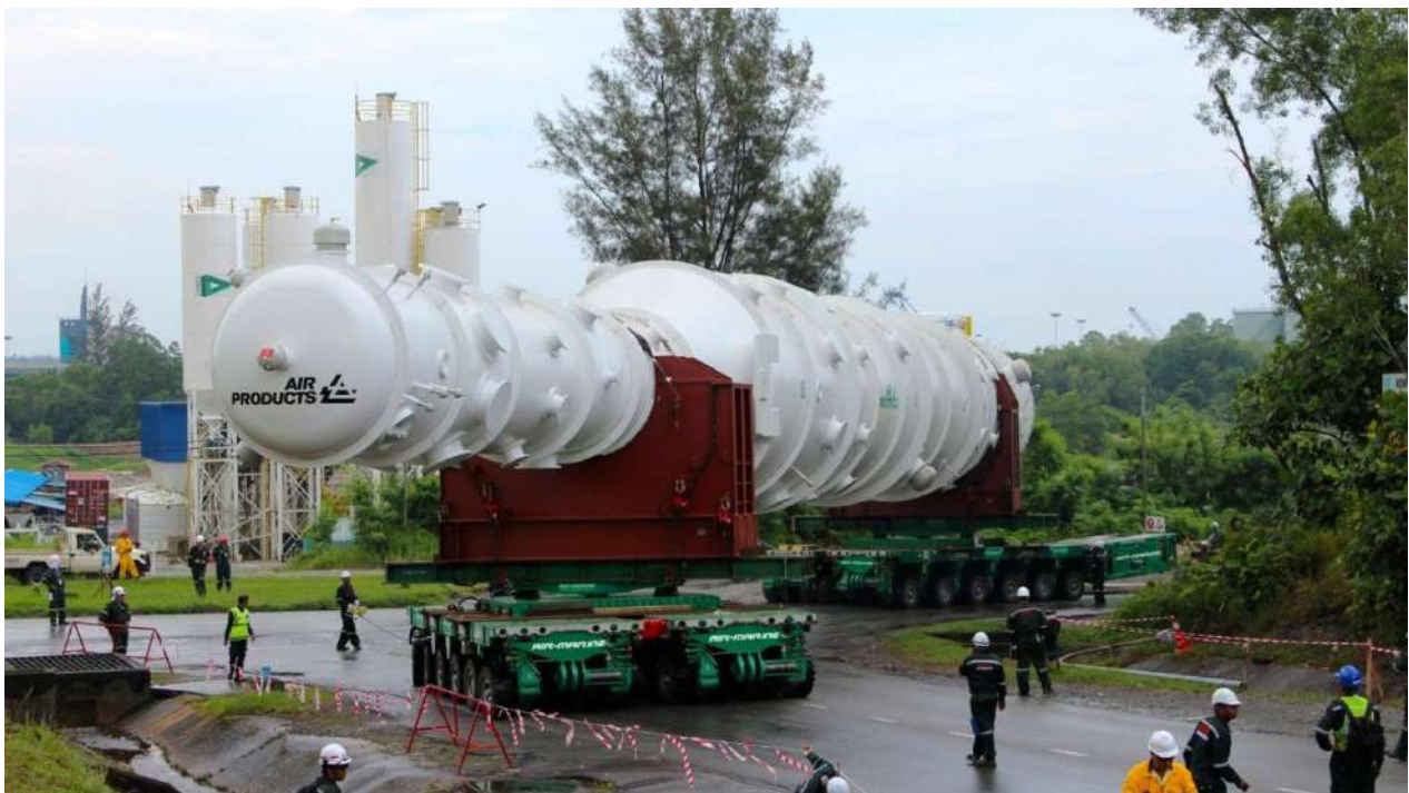
On 11th May 2014, AIR-MARINE transported a 300Te - 56m long, 5.4m wide and 6.1m high - Main Cryogenic Heat Exchanger (MCHE) from the port of Bintulu were assembled in 6 axeline in 4-file (side by side/double) in Dolly configuration, c/w 300Te Bolsters (Turntables) and a 350kW Diesel Driven Powerpacks on each 4-file system. In total there were 24 axelines SPMT's + 2PPU's + 300Te Bolsters which were utilised for the entire transport operation.
