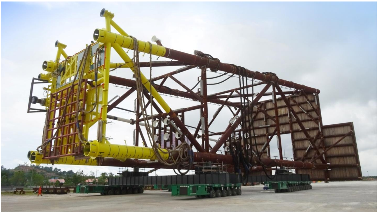
Shifting of 766Te BP-A (Bunga Pakma – A) Jacket by utilising our 36 axlelines of Scheuerle 4th Gen. Self Propelled Modular Trailers (SPMT's) coupled with 4units hydraulic Powerpack units from the fabrication area to the quayside for our prestigious and distinguished clients Oceannight Sdn Bhd on the 16th of August 2017, at their fabrication yard in Kuching, Sarawak, for Repsol Oil & Gas Malaysia Ltd. The synchronised shifting operation lasted for around one hour and subsequently upon reaching the quay side, the Jacket was loaded out to the already pre-ballasted 330' flat top ballastable barge by utilising 20nos of our diesel driven ballast pumps.
