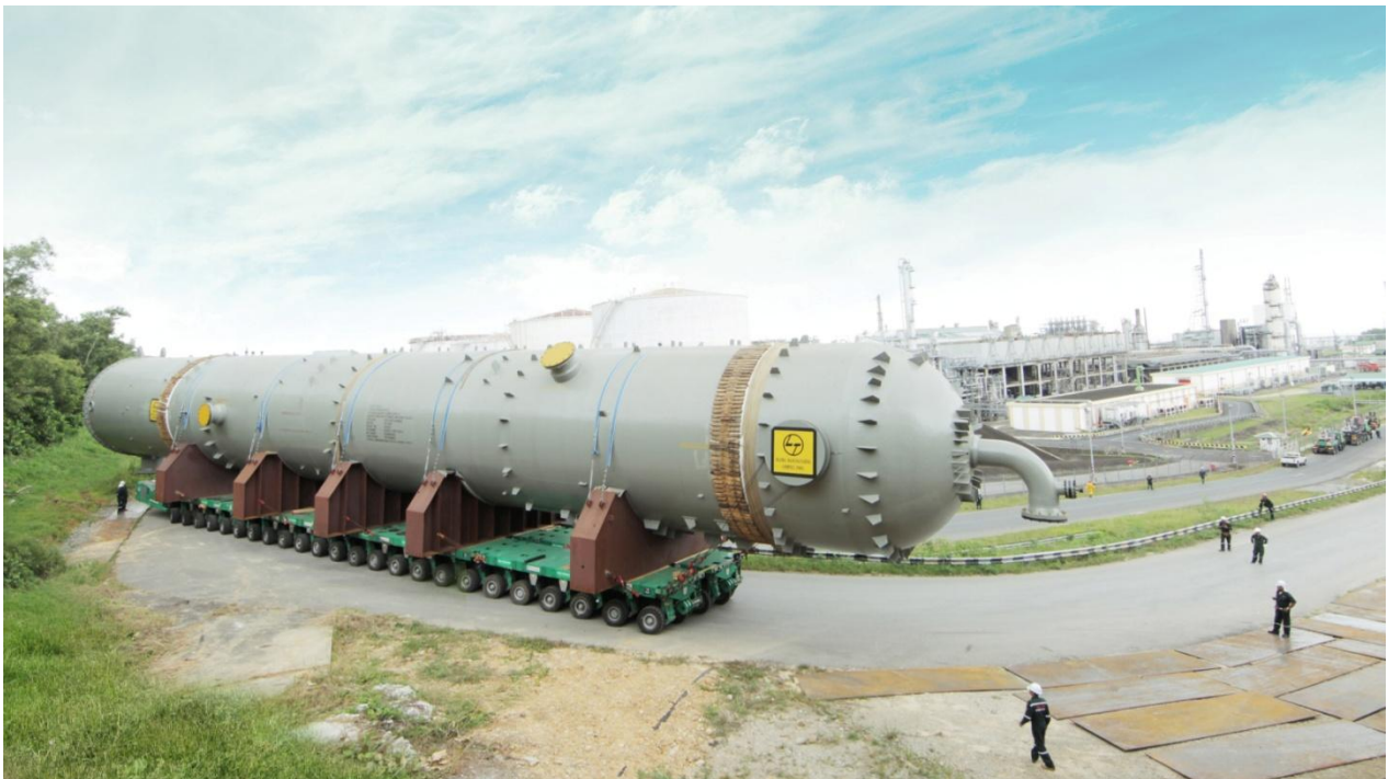
The successful accomplishment of heavy lift transportation for one (1) unit of Deep AGR Absorber Column for Petronas-MLNG with a combined weight of 1480 metric ton hauled from Bintulu Port to Petronas MLNG – Train 9 project site using 48 axle line SCHEUERLE Self Propelled Modular Transporter (SPMT). The sophisticated state-of-the-art equipment, excellent teamwork, cooperation and expert transport engineering have contributed to the success of this move on public road unmatched by any others in Malaysia.
