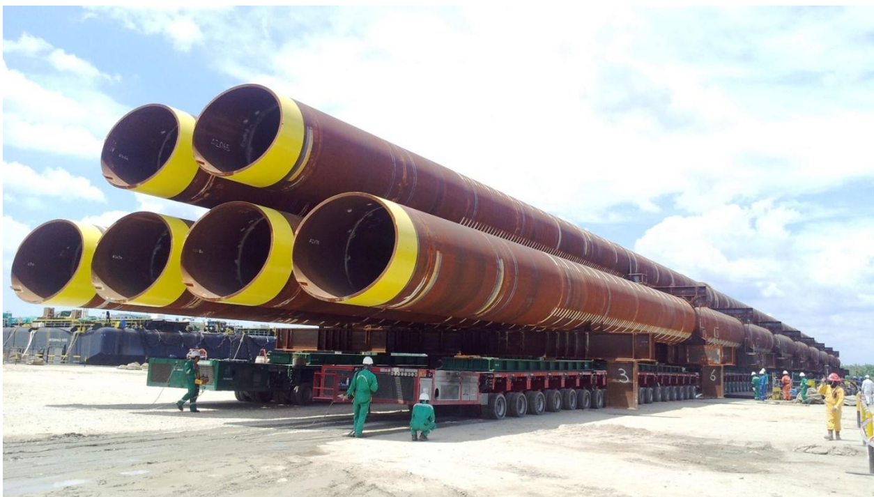
AIR-MARINE was contracted to load-out piles for KHL and KPOC from the fabricator's yard onto a barge. The 146 meter length and 3,582 tons weight of the pile set a record for the second longest and heaviest load-out in the world. We did this remarkable job using our 156 axle-lines of multi-axle trailers and 8 PPU. The combined transport weight was above 4300t. AIR-MARINE did load-out of 2 set of piles for this project.
