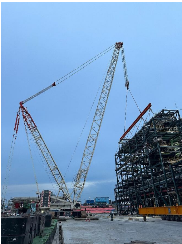
Transportation of 184T Module from Samalaju Port to OCI ME1 Samalaju Plant utilising SCHEUERLE SPMT 30 x 2 (60) axleline and 2 PPU. Using 800T DEMAG CC3800-1 with Boom Booster lifting Module + Accessories with a total load of 282T on top of another Module for the final installation.
