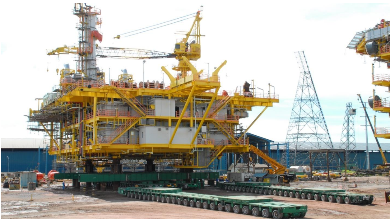
Shifting, Weighing, Loadout and Barge Ballasting for Sabah SHELL's St. Joseph Redevelopment Project's Water Injection Topside Module with combined weight 3000 tonnes for our esteemed client Brooke Dockyard And Engineering Works Corporation utilizing AIR-MARINE's 124 axle lines Goldhofer Self-Propelled Modular Transporter at Brooke Dockyard Fabrication Centre, Kuching, Sarawak, Malaysia on 3rd October 2010.
