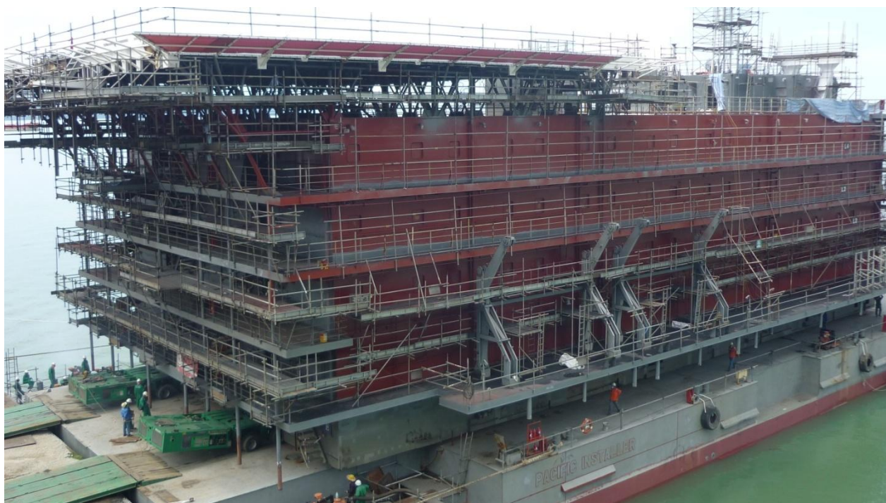
Shifting and Load out of a 2000 MT Accommodation Unit (H-131) onto a 111m Accommodation Barge in Boustead Penang Shipyard (BPS), Pulau Jelajak, Penang on 21 May 2011. A total of 2 x 36 - axle lines single file of Goldhofer THP combined with PST Self Propelled Hydraulic Controlled Modular Transporter.
