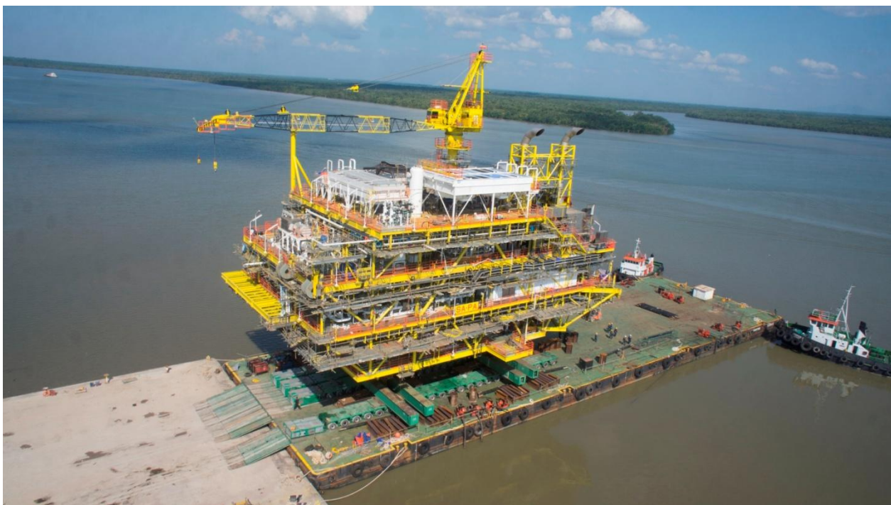
The SA-PA Topside weighing 2408MT was fabricated at BDEWC yard in Kuching, Sarawak for Murphy Sarawak Oil Co. Ltd. AIR-MARINE utilised 96 axle lines of Self-Propelled Modular Trailers and 4 power packs to transport and loadout the structure to barge 'Maritime Courage'. 16 units of deck pumps were used for the ballasting / deballasting works during the loadout. AIR-MARINE also provided 4x27m loadout beams, 15 units of RO-RO Ramps and 30 units of wooden wedges required for the loadout operation.
