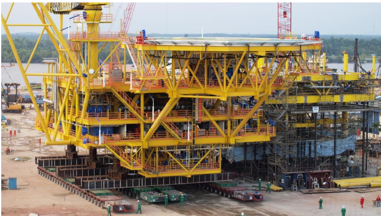
Shifting and Loadout of F28 DR-A TOPSIDE at Kencana HL Yard, Lumut; a project by Shell Berhad, on 21st-22nd June 2011. A total of 2 x 24 axles SLE and 2 x 12 axles ESE (72 axles Goldhofer trailers) were used to transport the topside weighing almost 2224 tonnes. The topside was shifted at a distance of 400 meters before crossing over to the barge the following day. 14 ballast pumps were used for ballasting.
