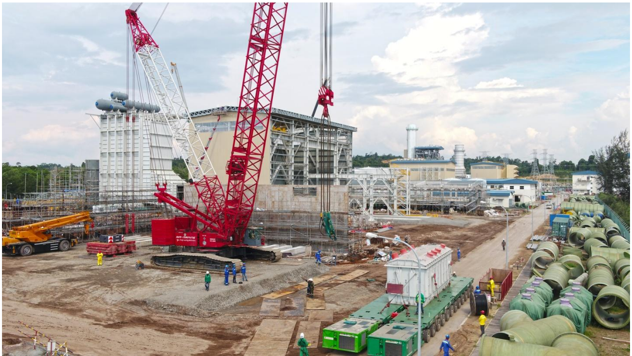
Transportation of transformer from Bintulu Port to TKCCPP Site using 24 axeline SCHEUERLE 4 th Generation SPMT and lifting of Transformer using Demag CC2600
