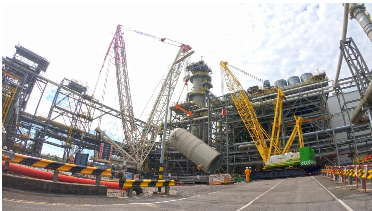
Transportation of Absorber Column from Bintulu Port to MRU Project Site using 10 + ½ PST/THP Goldhofer trailer and lifting utilising Demag CC3800-1
