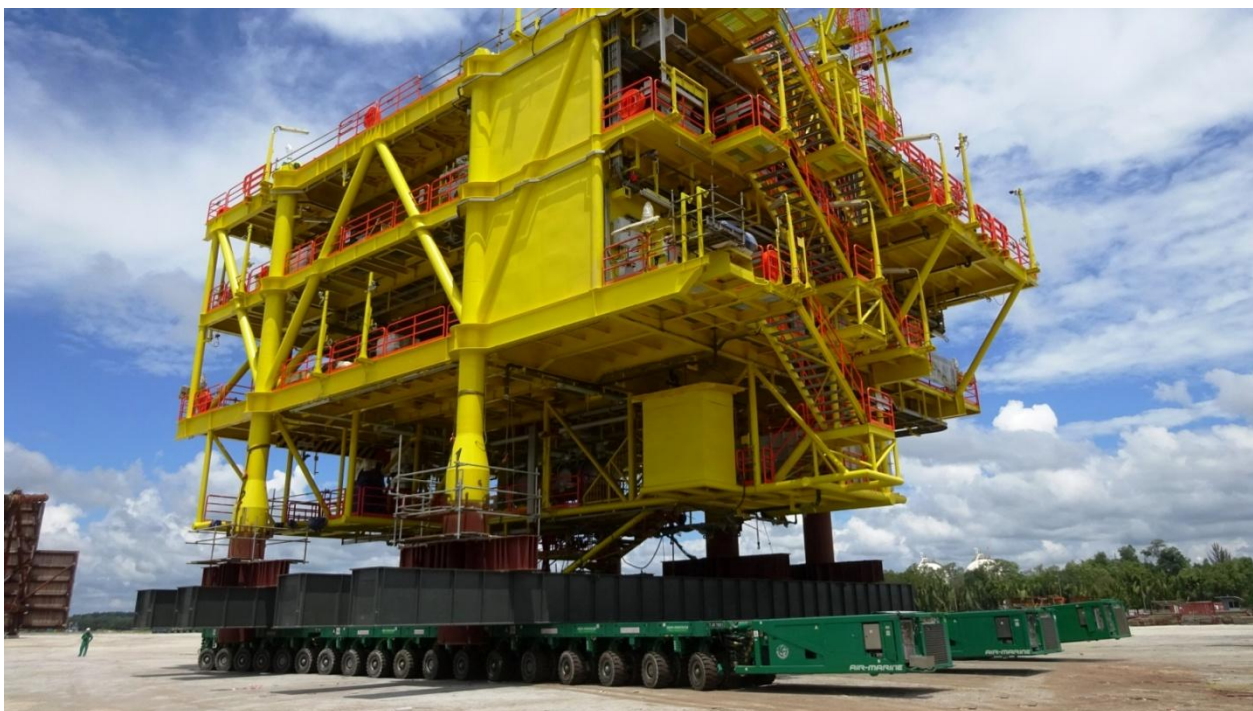
Shifting of 812Te BP-A (Bunga Pakma – A) Topside by utilising our 54 axelines of Scheuerle 4th Gen. Self Propelled Modular Trailers (SPMT's) coupled with 3units hydraulic Powerpack units from the fabrication area to the quayside for our prestigious and distinguished clients Oceanright Sdn Bhd on the 11th of August 2017, at their fabrication yard in Kuching, Sarawak, for Repsol Oil & Gas Malaysia Ltd. The synchronised shifting operation lasted for around one hour and subsequently upon reaching the quay side, the Topside was loaded out to the already pre-ballasted 330' flat top ballastable barge by utilising 20nos of our diesel driven ballast pumps.
