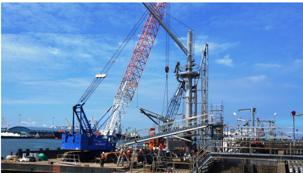
Erection of Sarawak SHELL Berhad's Loading Arm weighing 50 MT utilizing Hitachi KH500 as main crane and Kobelco 7450 as tailing crane.
