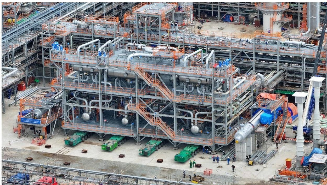
✓ Load-in operation of 840 MT module from MOLF jetty at Bintulu utilizing 30 x 2 axleline and 2 PPU SPMT and transport to OGP site. Upon arrival, the configuration of the SPMT changed to 18 x 4 axleline and 4 PPU to manoeuvre into the highly congested area. The final installation is completed by jacking down onto permanent support ensuring perfect alignment and load transfer to the foundation.
