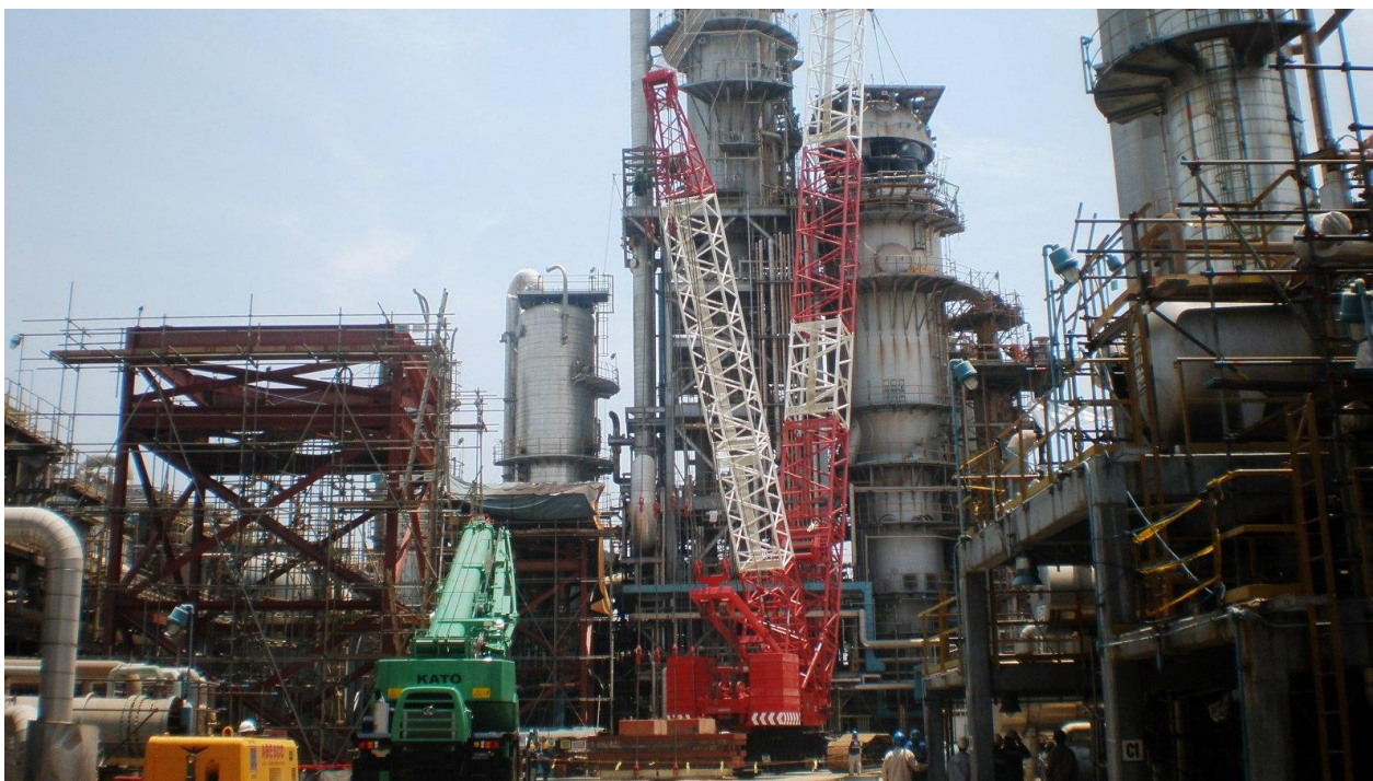
Provision of one (1) unit 600-Ton Demag CC2600 Crawler Crane at Limay, Bataan, Philippines for lifting one (1) unit Cyclone Assembly weighing 165 MT, with dimension of 7.6m(D) X 12m(H) and lifting height of 55m at Petron Refinery.
