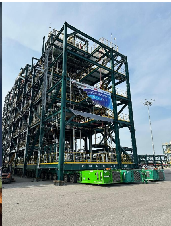
Load-in operation of 826T Module (L38 x W12 x H34m) from Samalaju Port to OCI ME1 Samalaju Plant utilising SCHEUERLE SPMT 36 x 3 (108) axleline and 3 PPU. The final installation is completed by jacking down onto Site Foundation through Gen 4 SCHEUERLE wireless remote system ensuring precision control.
