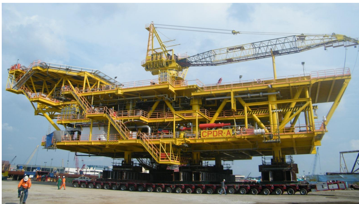
Shifting and loadout of CPDR-A Topside weighing 1958 MT for Cili Padi Gas Field Development Project at Kencana Yard, Lumut utilizing 72 axles Goldhofer PST-SLE and PST-ESE Electronic Multiway Steering System Modular Transporter on the 19th September 2010. Ten (10) units of ballast pump were used on the offshore barge to maintain stability during the cross-over.
