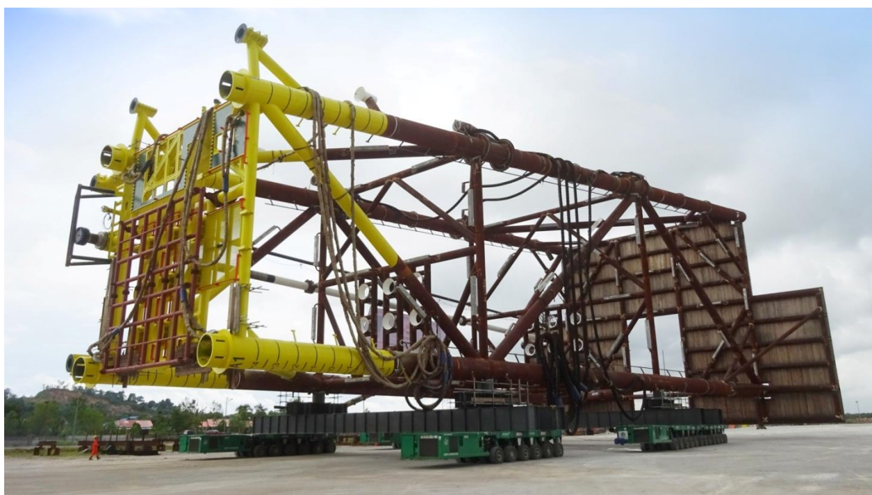
Shifting of 766Te BP-A (Bunga Pakma – A) Jacket by utilising our 36 axles of Scheuerle 4th Gen. Self Propelled Modular Trailers (SPMT's) coupled with 4 units hydraulic Powerpack units from the fabrication area to the quayside for our prestigious and distinguished clients Oceanright Sdn Bhd on the 16th of August 2017, at their fabrication yard in Kuching, Sarawak, for Repsol Oil & Gas Malaysia Ltd. The synchronised shifting operation lasted for around one hour and subsequently upon reaching the quay side, the Jacket was loaded out to the already pre-ballasted 330' flat top ballastable barge by utilising 20nos of our diesel driven ballast pumps.
